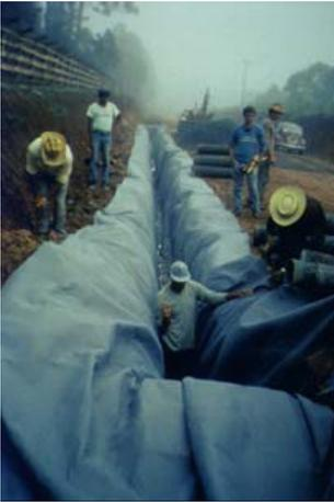
The filter has also to be considerably more permeable than the base soil throughout the project life time. Therefore, the permeability criterion for geotextiles establishes that
