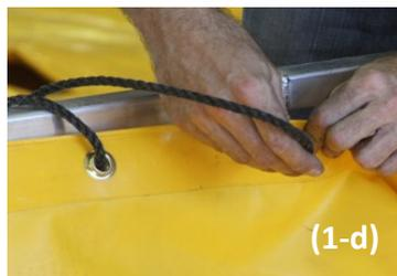
**Step 3:** Unfold the tank. Ensure that the tank liner is not pinched or impeded by the frame.
