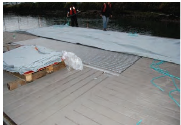
Barge Silt Curtain being Installed on Barge Deck
