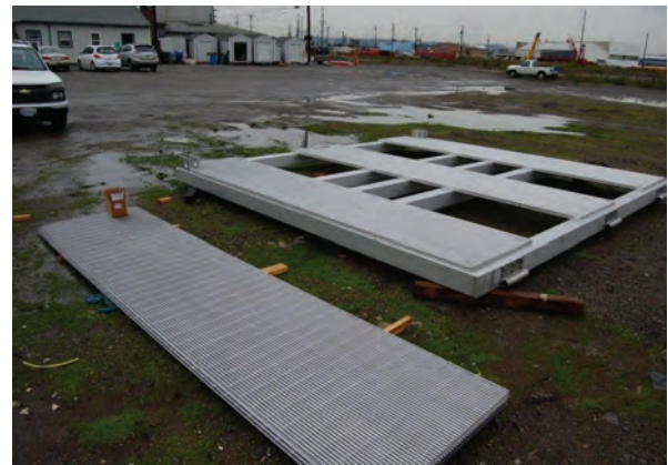
Barge Deck Being Produced
