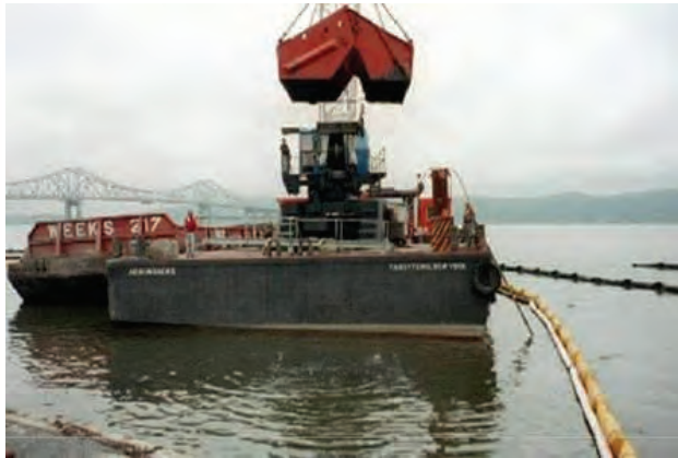
Silt Barrier being Installed
