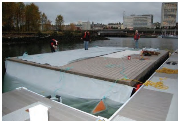
Barge Silt Curtain being Installed on Barge Deck
