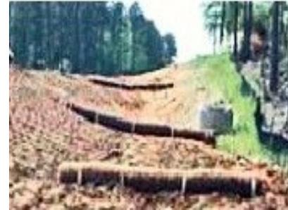
Coir Wattles are made from cleaned mattress coir fiber that has been lightly packed inside of a high strength bristle coir twine netting. With a lighter packing, these wattles leave enough room for clean water to pass through. This creates a system for controlling your erosion and filtering out sediment from your area. Wattles are frequently used in both construction & landscaping projects.
