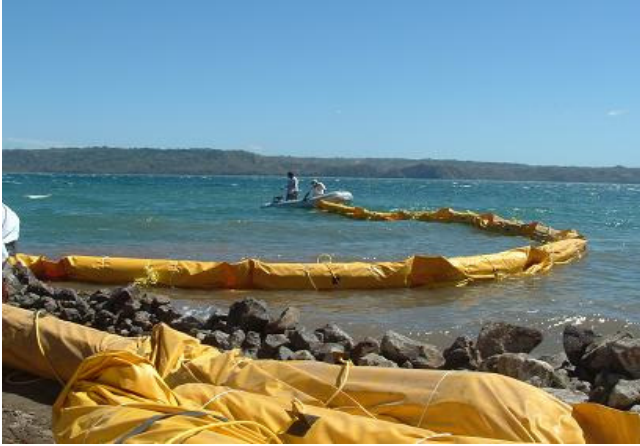
Deploying Silt Curtain with Small Boat
