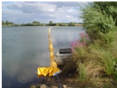
Type 2 Silt Barrier in Action
