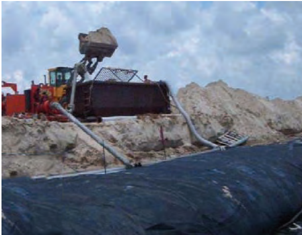
Slurry/Sand Mix Preparation & Pump Running
