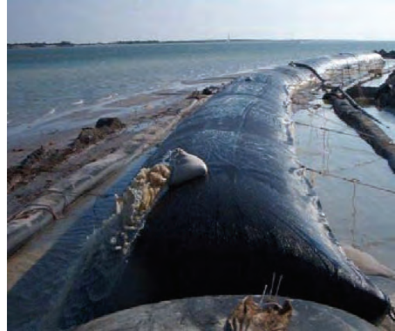
Installed Breakwater Tubes
