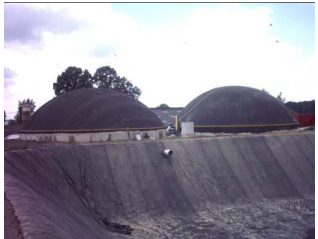
Anaerobic digesters with waste lagoon
